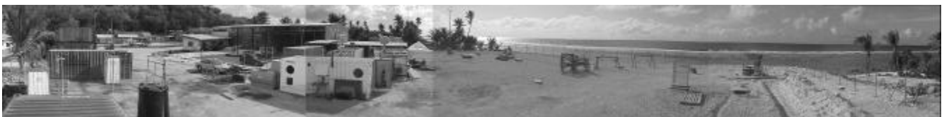
Figure 5. Panoramic view of site looking southeast to northwest (left to right).
